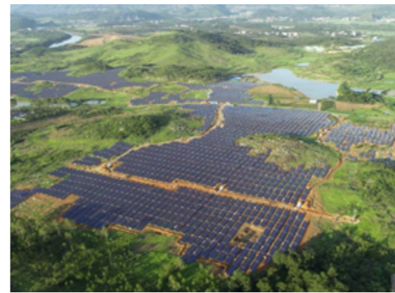
Poverty Alleviation PV Power Station in Jianghua Yao Autonomous County, Hunan Province
